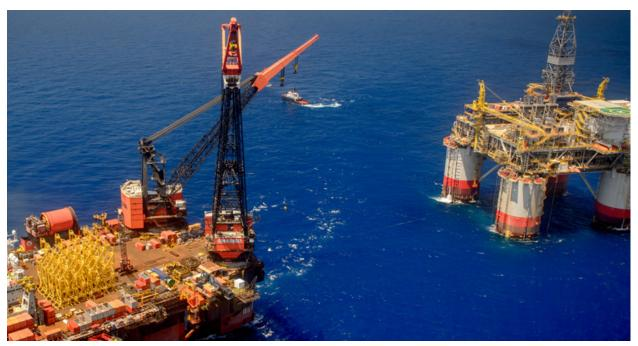
Big Foot is a dry-tree Extended Tension-Leg Platform (ETLP) with an on-board drilling rig and production capacity of 75,000 barrels of oil and 25 million cubic feet of natural gas per day. The Big Foot field was discovered in 2006 and is estimated to contain total recoverable resources in excess of 200 million oil-equivalent barrels. Chevron estimates the field will be in production for approximately 35-years.
