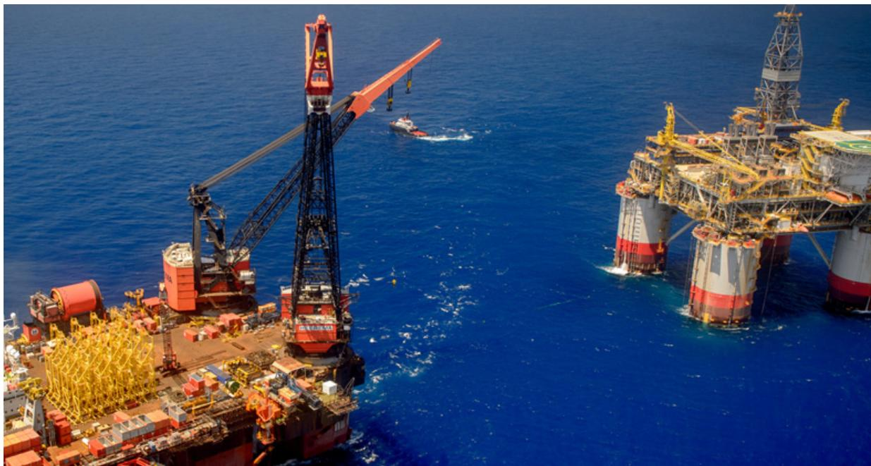
*Big Foot is a dry-tree Extended Tension-Leg Platform (ETLP) with an on-board drilling rig and production capacity of 75,000 barrels of oil and 25 million cubic feet of natural gas per day. The Big Foot field was discovered in 2006 and is estimated to contain total recoverable resources in excess of 200 million oil-equivalent barrels. Chevron estimates the field will be in production for approximately 35-years.*
